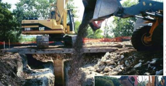
The biowalls were excavated with a hydraulic excavator (shallow trenches) or rock-trencher (deep trenches) and backfilled with a mixture of mushroom compost, pine wood chips, soybean oil, and limestone aggregate. Diffuser pipes were installed on the bottom of each trench to allow for future injections of soybean oil or other carbon substrates as needed.
